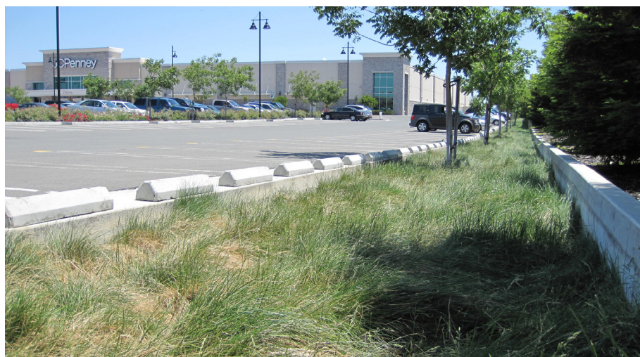
This bioretention facility provides stormwater treatment and flow duration control for a big-box retail store in Antioch.
